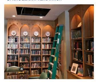
The Property Committee is overseeing the renovation of the Ziegler Adult Library this Spring. The tile ceiling will be removed to expose the beaded and beam wooden ceiling that is on the east two-thirds of the room and will be replicated on the remaining ceiling along with new LED lighting and heat/air conditioning. The carpet will be removed, and a new floor installed. The use of the room will be expanded to include a chapel space for intimate worship gatherings.
