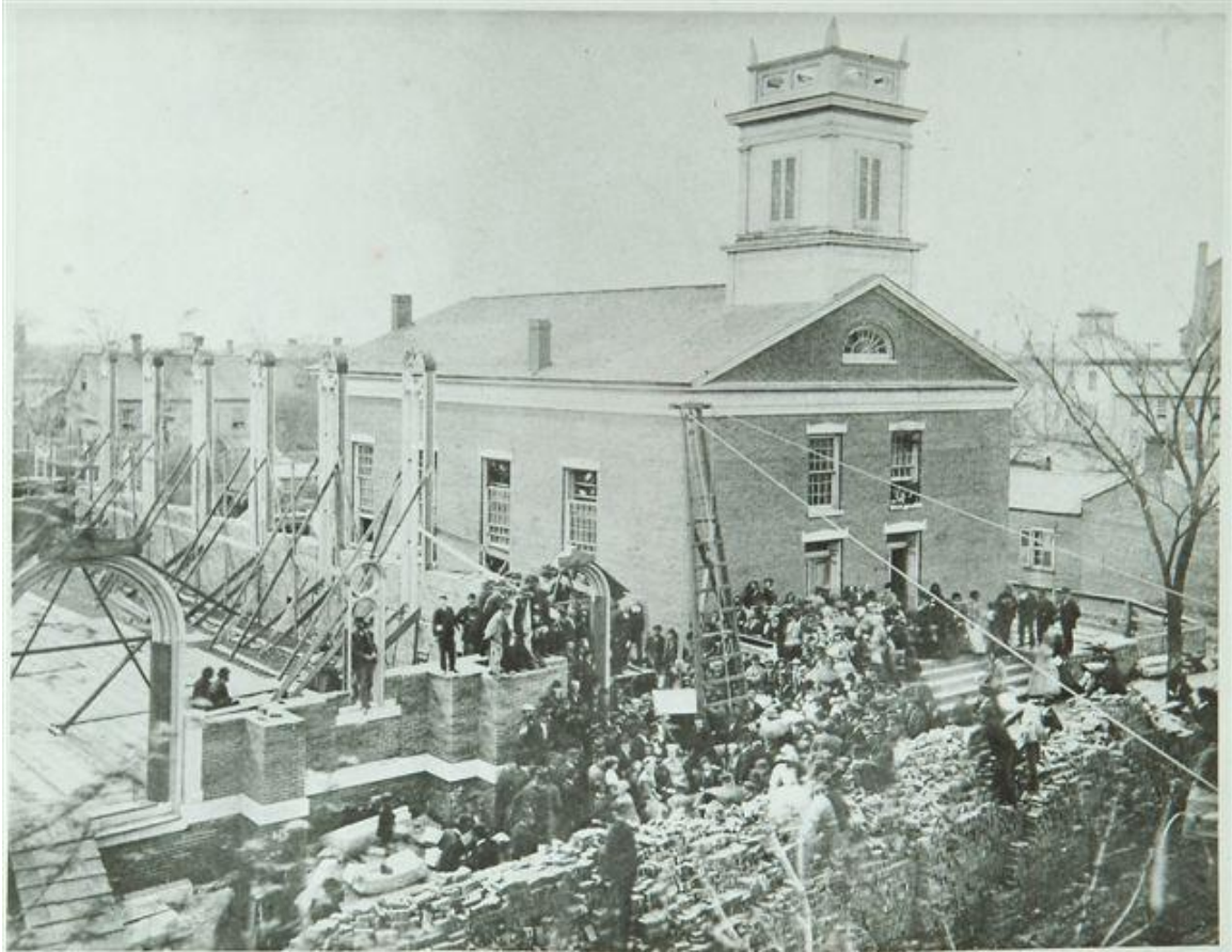
Laying the Cornerstone 1869
